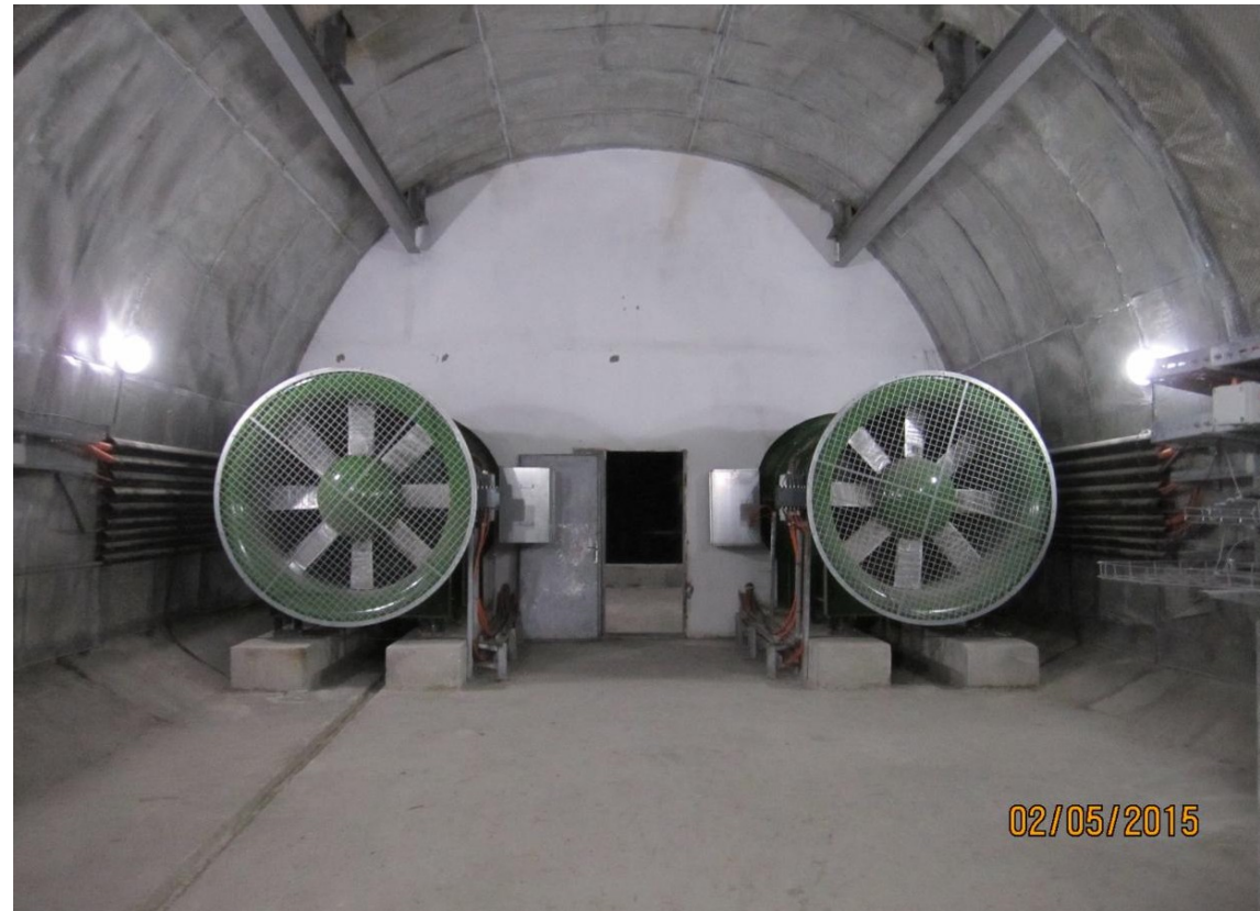
Picture of metro fan commissioning
