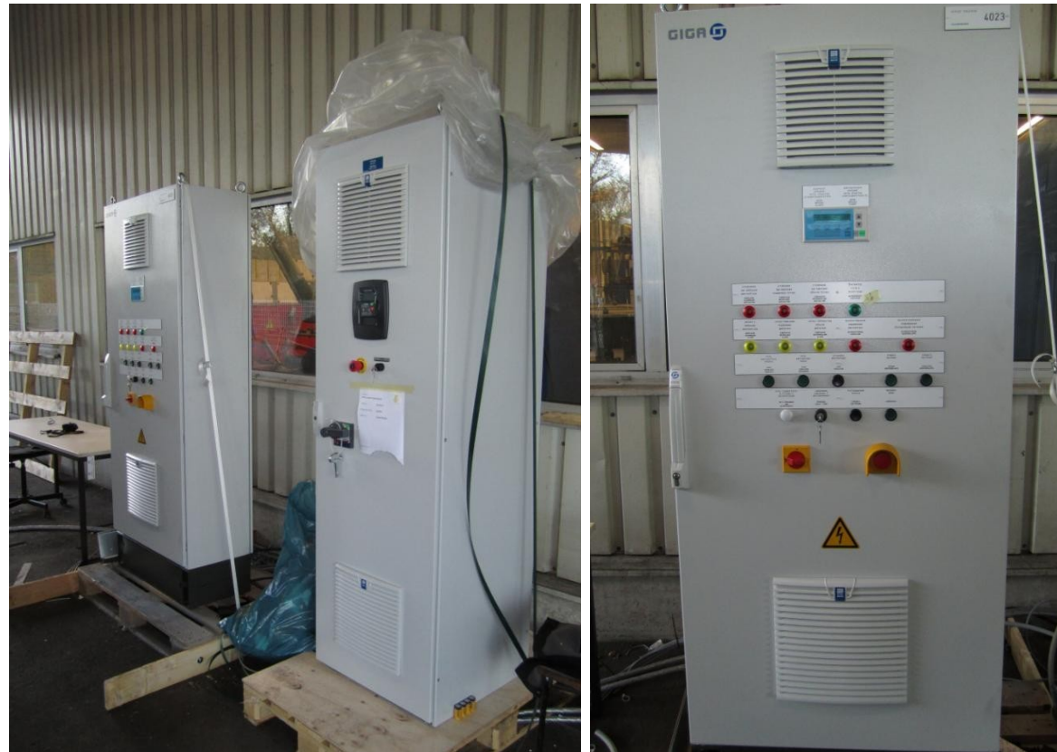
Picture of VSD & control panel for Metro Almaty
