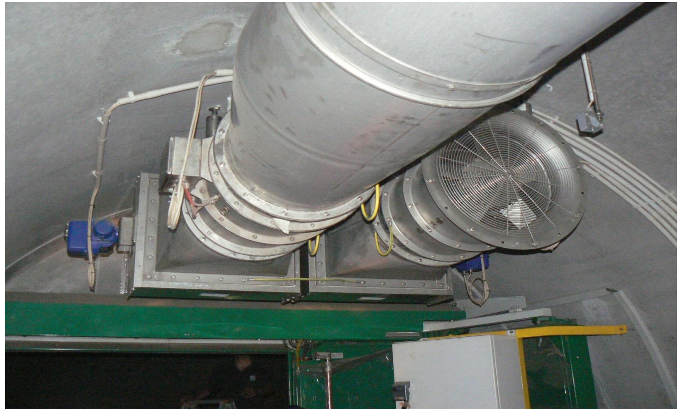
Picture of over pressure fans
