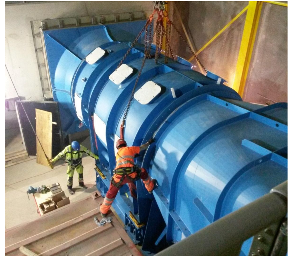
Pictures of fan installation
