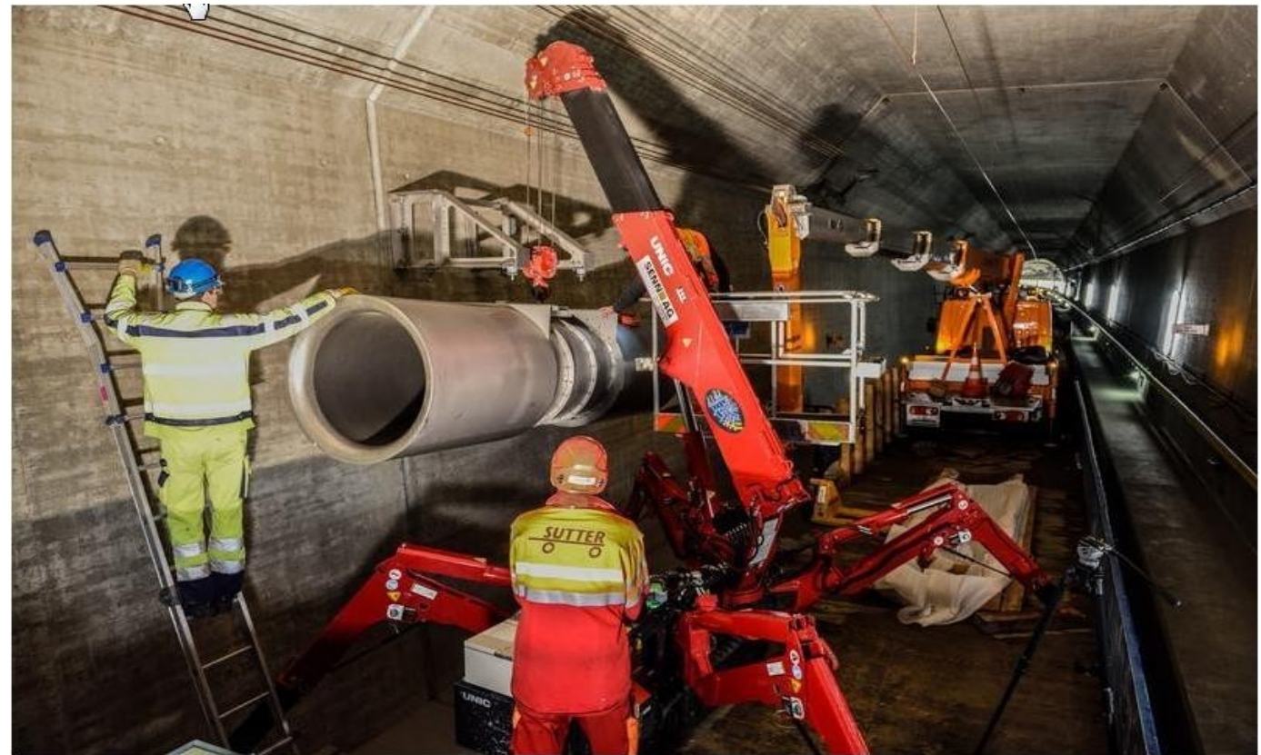
Picture of Jet Fan installation
