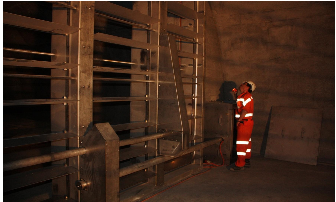
Picture of exhaust air hatch
